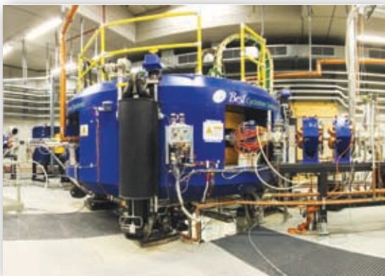
Installation of Best™ 70 MeV Cyclotron at INFN, Legnaro, Italy
